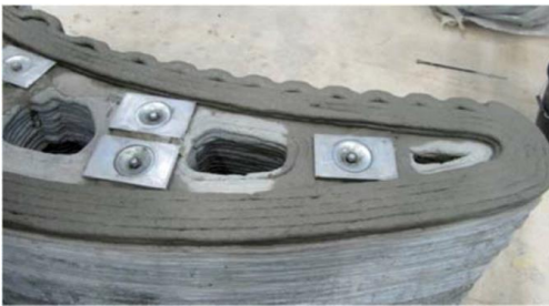
Post-tensioning of steel reinforcement placed in 3D printed conduits
