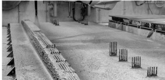
Concrete floor slabs with add-on-printed reinforced ribs
