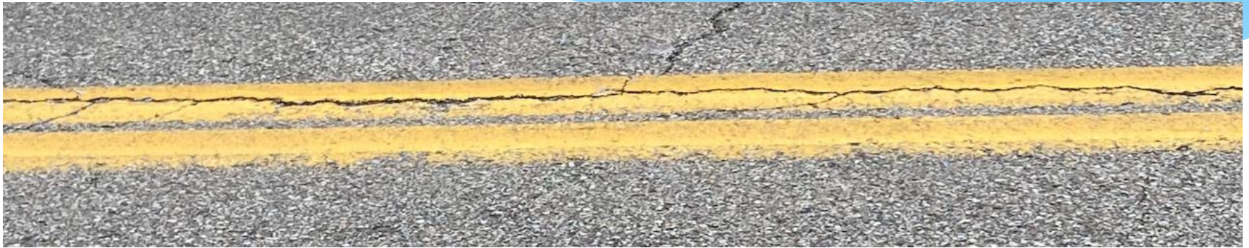
Deteriorated Joint
