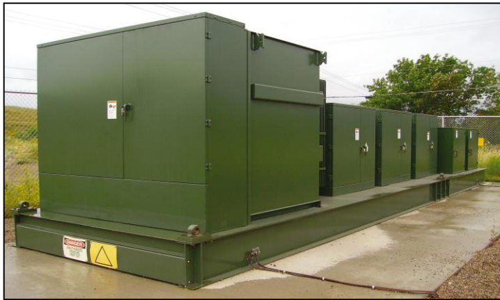
Modular Integrated Transportable Substation (MITS)
