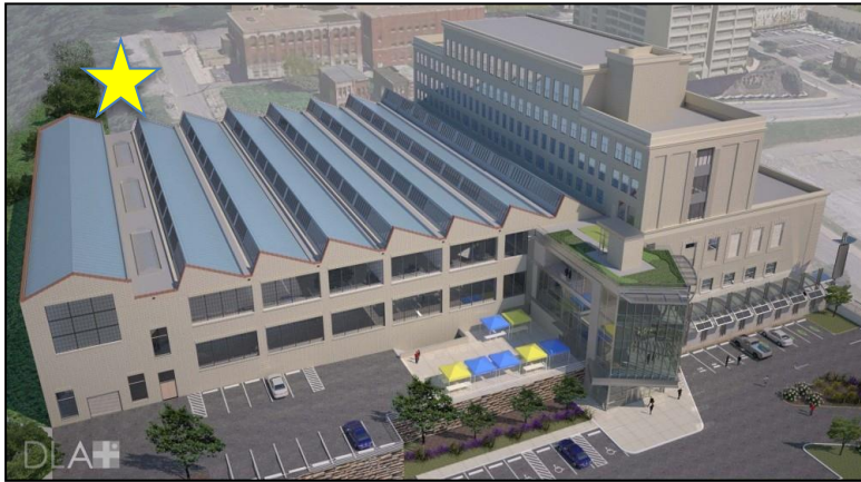
Outdoor Location of HV Interconnection – MITS
