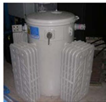
330kVA 60Hz Transformer 55" high and 2700Lb
