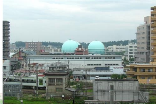
SAIWAITYOU NATURAL GAS FACILITY
