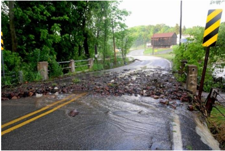
Debris on road
