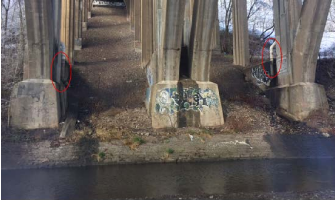
Figure 4.2 Drainage pipe from PennDOT bridge to NMR
