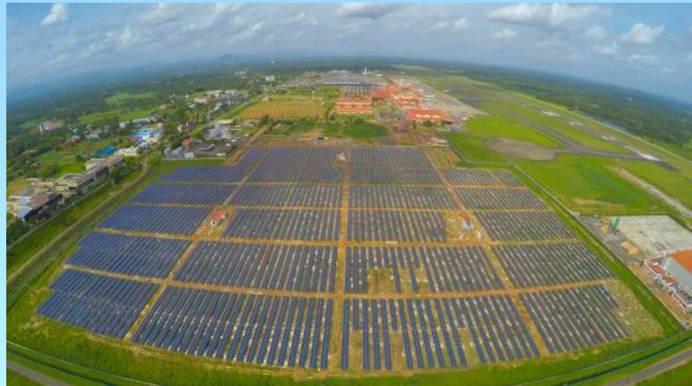
Cochin airport, 12 MW solar. www.thehindubusinessline.com
