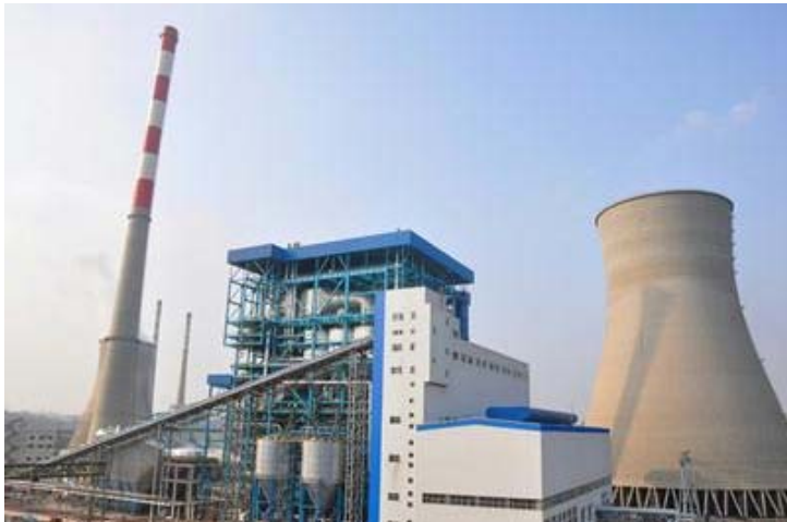
Shenhua Baima Circulating Fluidized Bed Boiler Power Station
