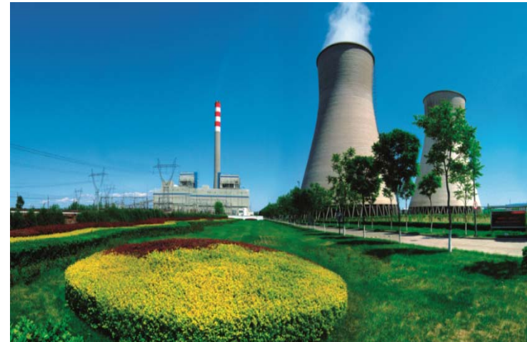
Shenhua Zhoushan Coal-fired Power Station
