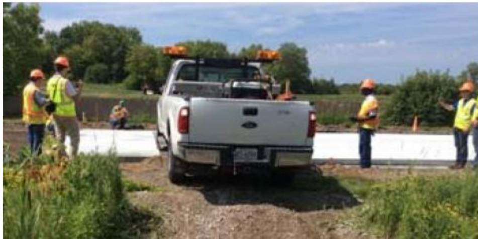
Loading 2 hours after paving
