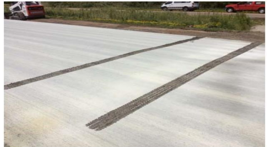
Loading 2 hours after paving
