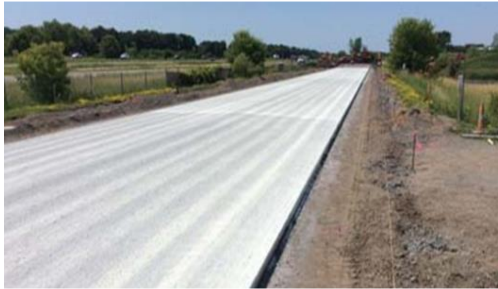
Loading 2 hours after paving
