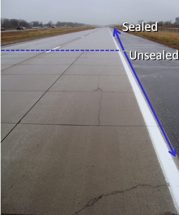
FIGURE 7 Companion test sections with sealed and unsealed joints.
