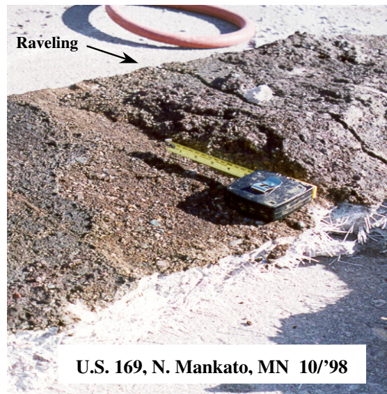
FIGURE 6 Three different modes of debonding between the HMA and concrete overlay.
