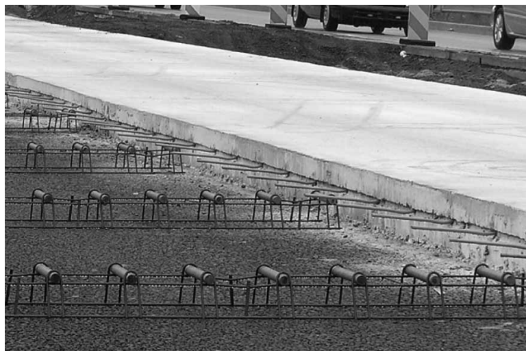
Figure 2. Dowel and tie bar configuration on SR-22.
