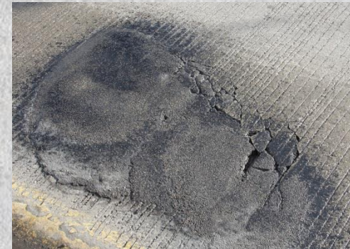
mortar patch of LMC ↑
