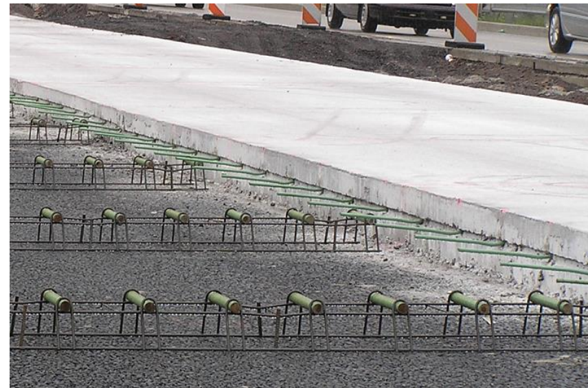
Dowel and tie bars in restrained section
