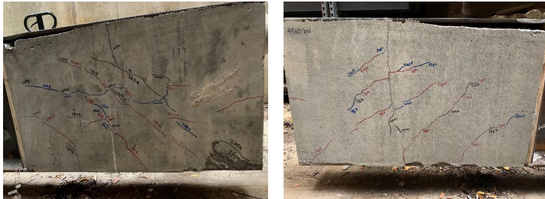
a) East side (support bearing at right)
