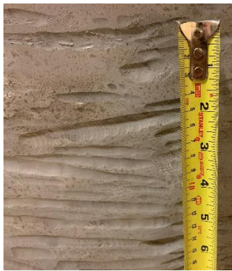
SSPC SP5 surface preparation
