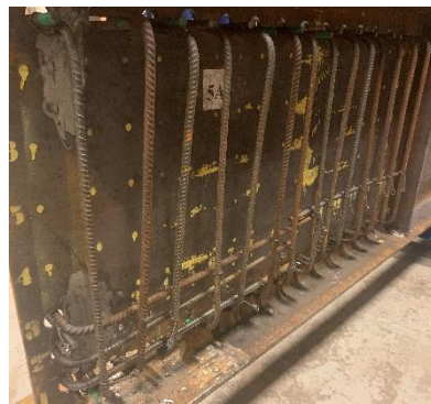
steel hairpins in place
