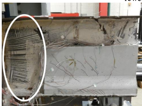
c) cracking of near side of UHPC panel (end of girder at right)
