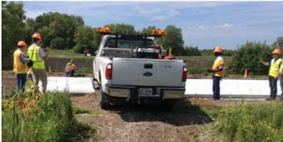
Loading 2 hours after paving
