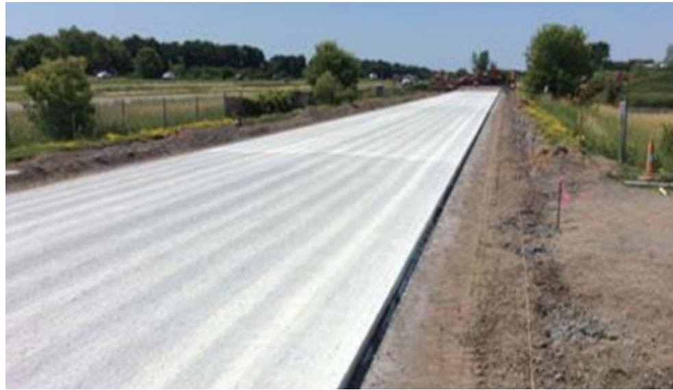
Loading 2 hours after paving
