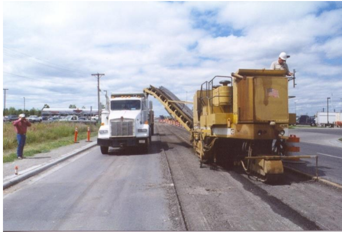
Figure 8. Milling prior to the placement of the PCC overlay.
