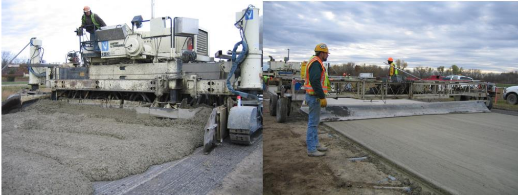
Figure 14. Paving and finishing an unbonded overlay.
