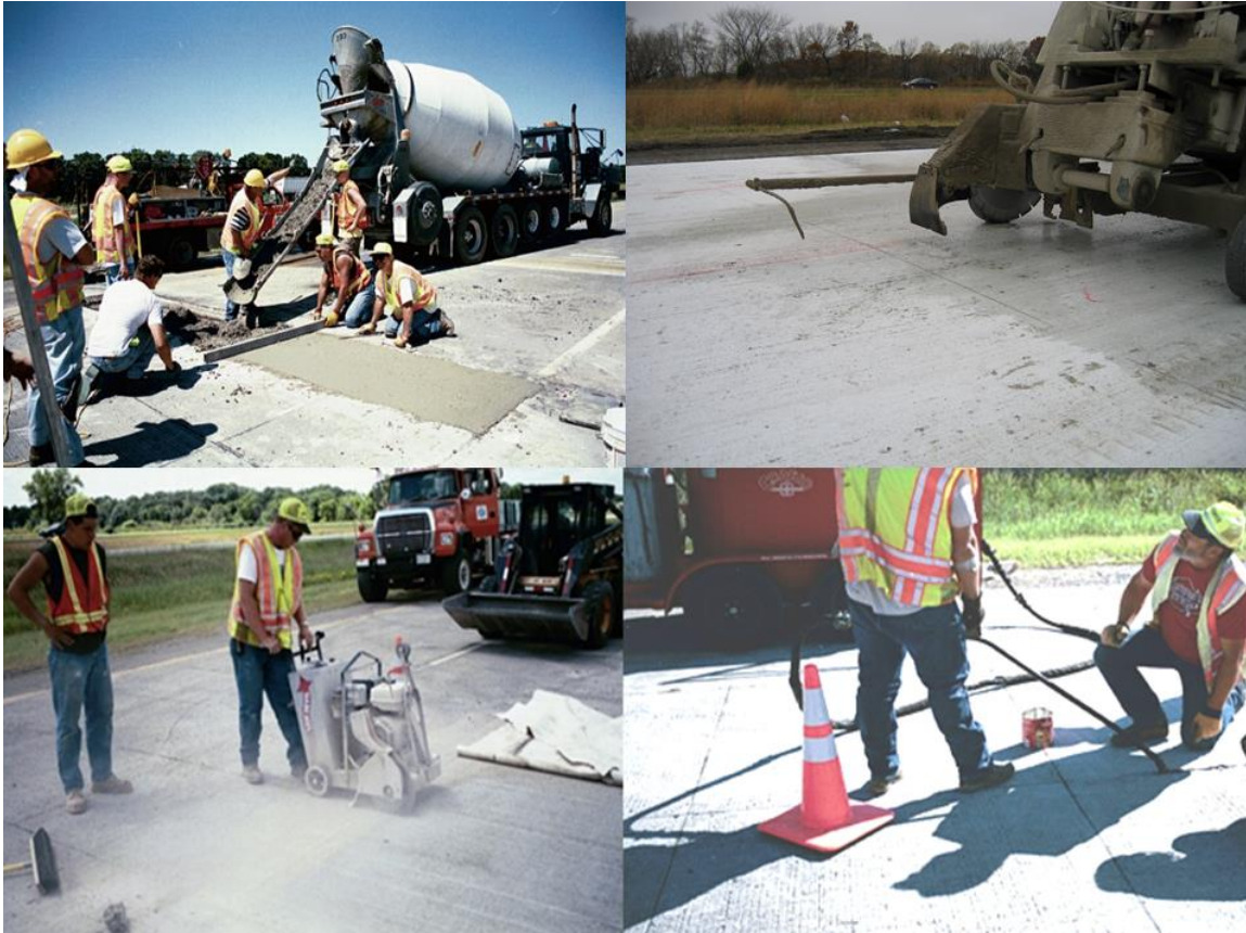
Figure 6. Placing the concrete in the repair and sawing and sealing.
