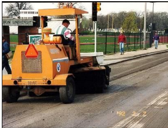
Figure 9. Sweeping the HMA surface after milling.
