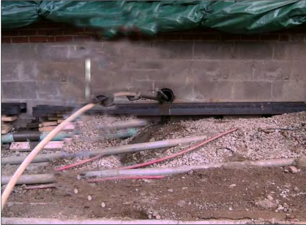
Figure 10-62 - Example Tremie Grout Placement for Tieback with Grout Tube, Allegheny County, PA
