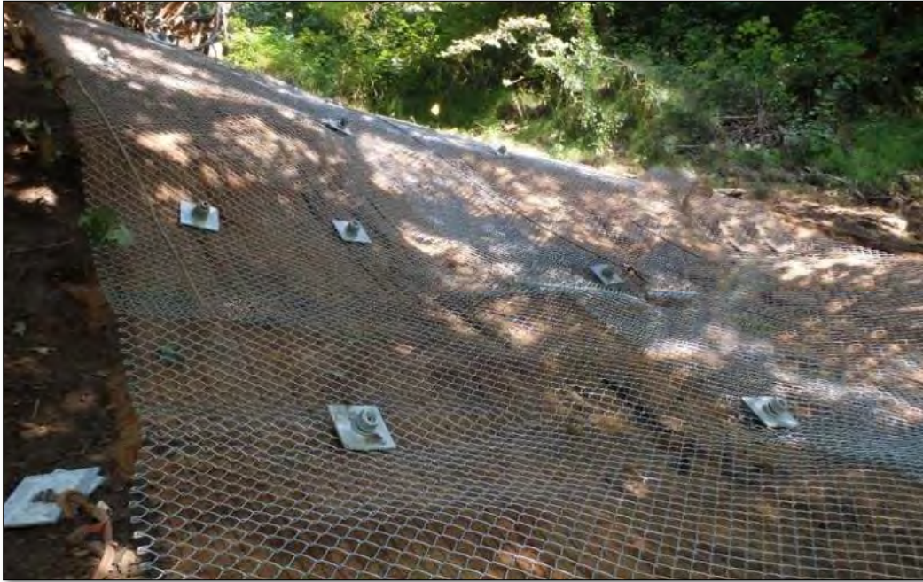
Figure 10-77 - Soil Nails and Wire Mesh
