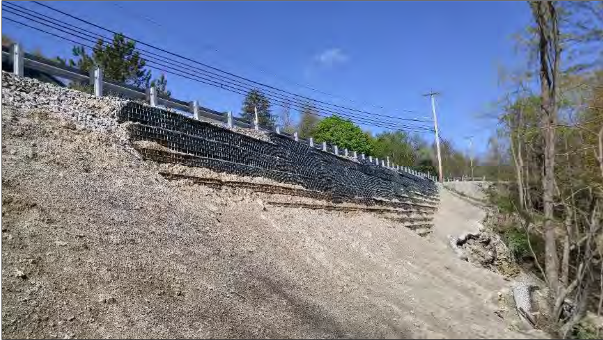
Figure 10-20 - GRS Slope (PennDOT District 11)
