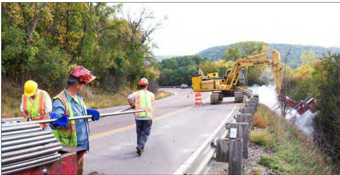
Figure 10-82 - Soil Nail Launcher [57]
