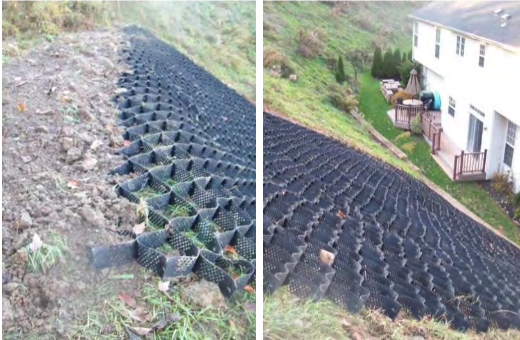
Figure 10-23 - Geocell Installation
