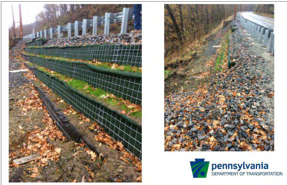
Figure 10-19 - Constructed GRS Slope Along a Roadway (PennDOT District 11)
