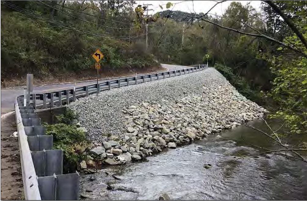
Figure 10-31 - Rock Slope (PennDOT District 11)
