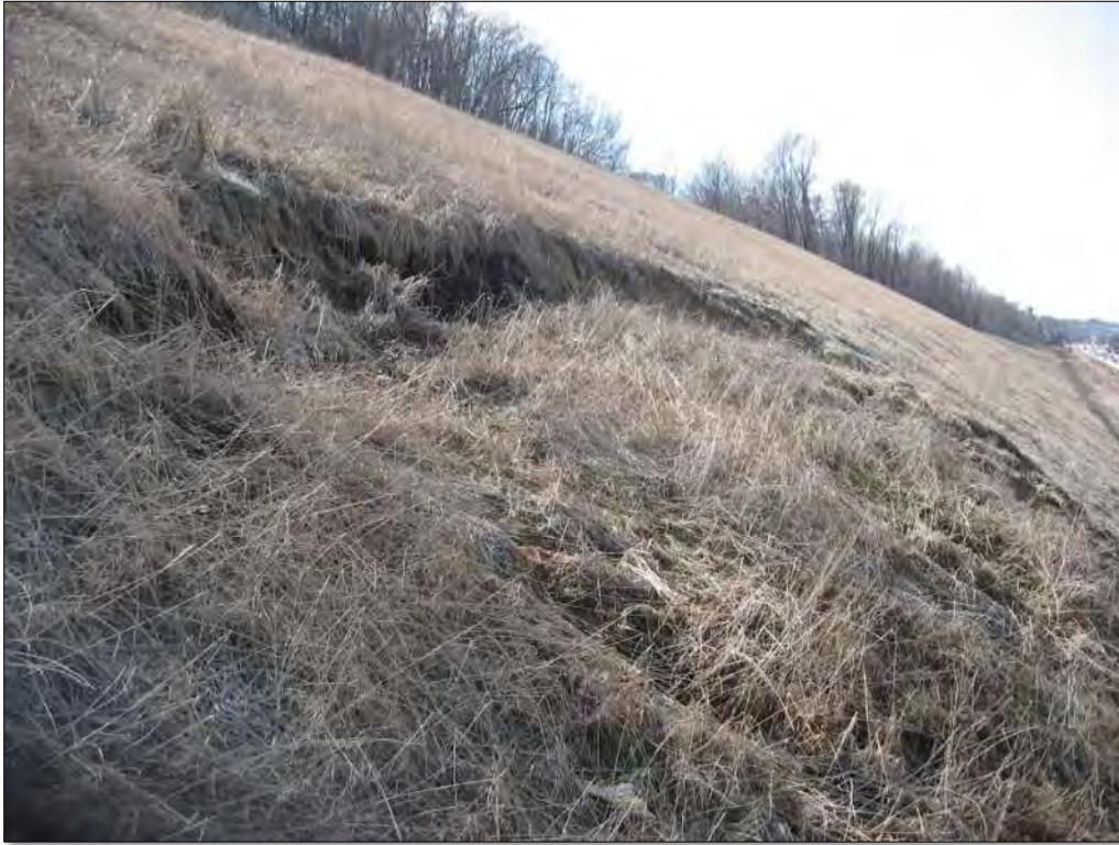
Figure 10-96 - Head scarp forming due to loss of shear strength from seepage
