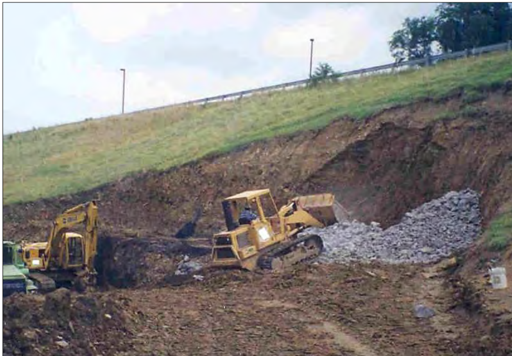
Figure 10-13 - Construction of Rock-Fill Buttress to Repair Landslide
