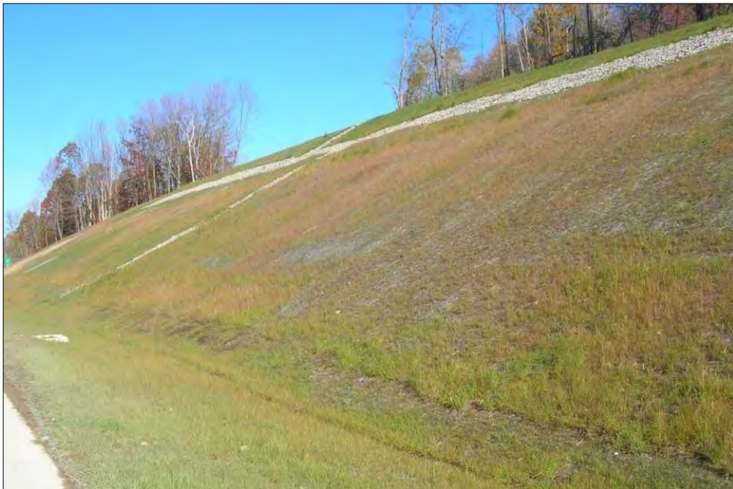
Figure 10-99 - Finger Drains on Slope
