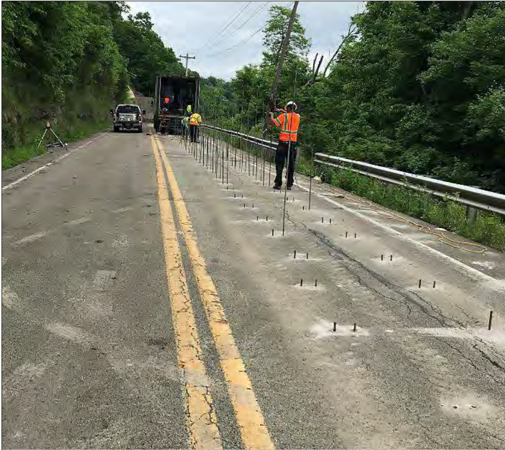
Figure 10-117 - Deep Polymer Injection, Fayette County, PA (PennDOT District 12)
