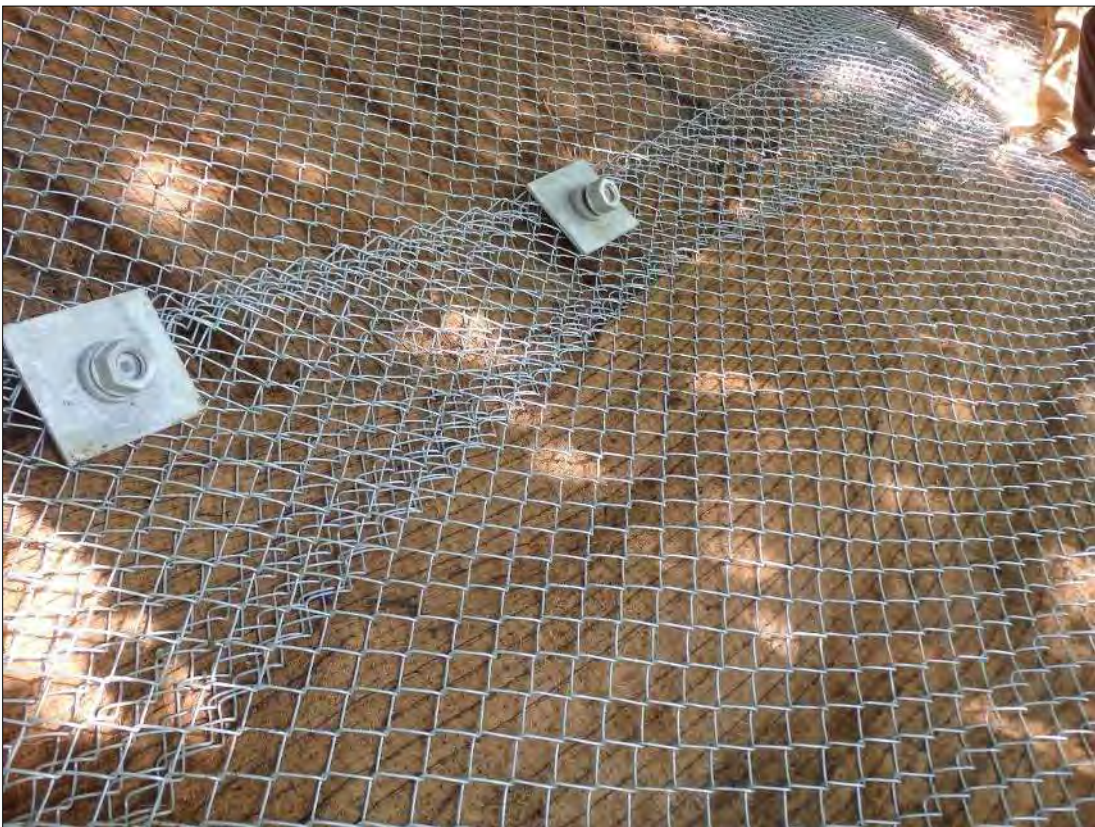
Figure 10-76 - Soil Nails and Wire Mesh
