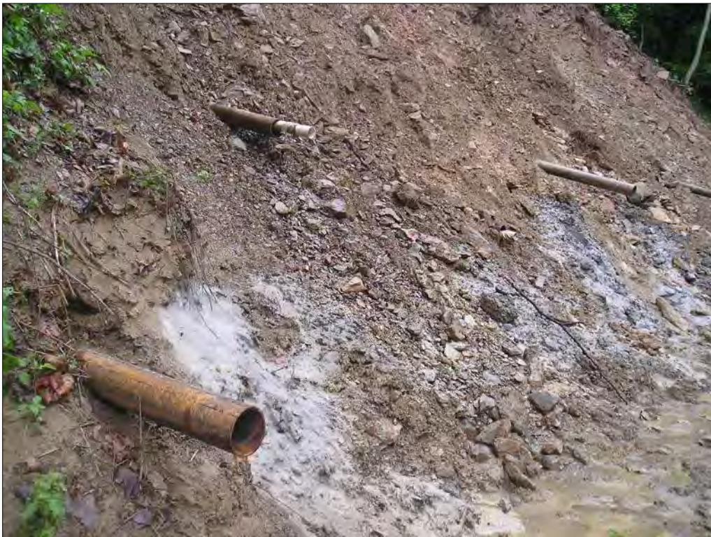
Figure 10-104 - Completed Horizontal Drains, Note Seepage Emanating Beside Surface Casing for Drain
