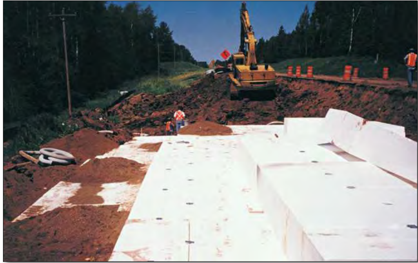
Figure 10-105 - Geofom for Landslide Repair [124]
