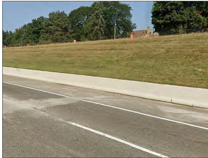
Figure 10-41 - Single-Face Barrier at Toe of Slope [60]
