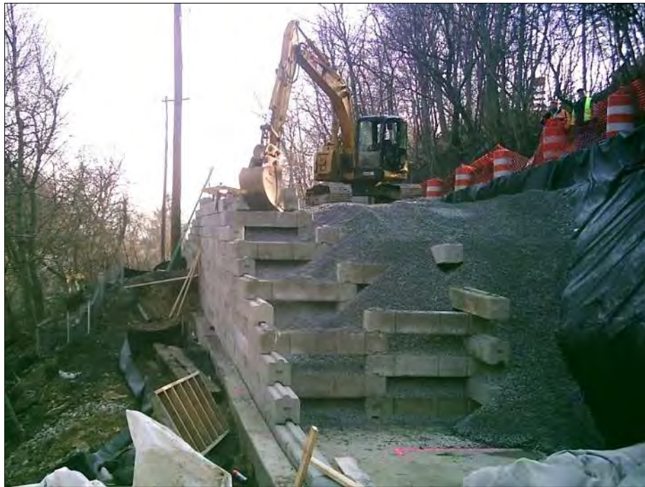
Figure 10-51 - Crib Wall Construction to Repair Slope and Support Road
