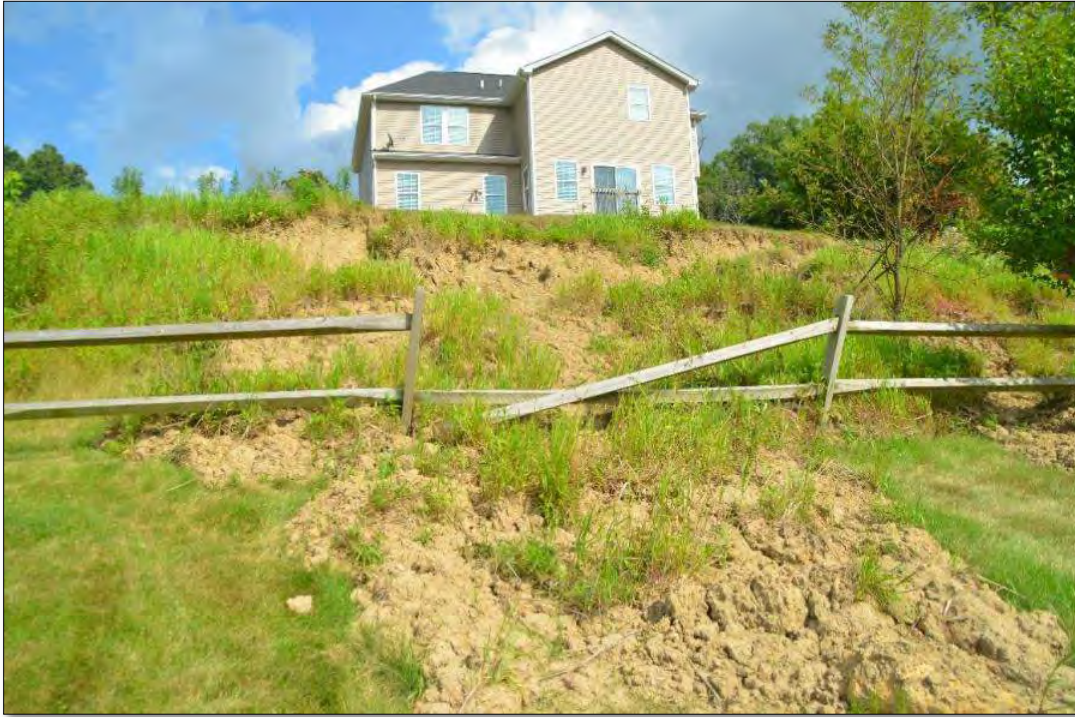
Figure 10-109 - Existing Rotational Slide
