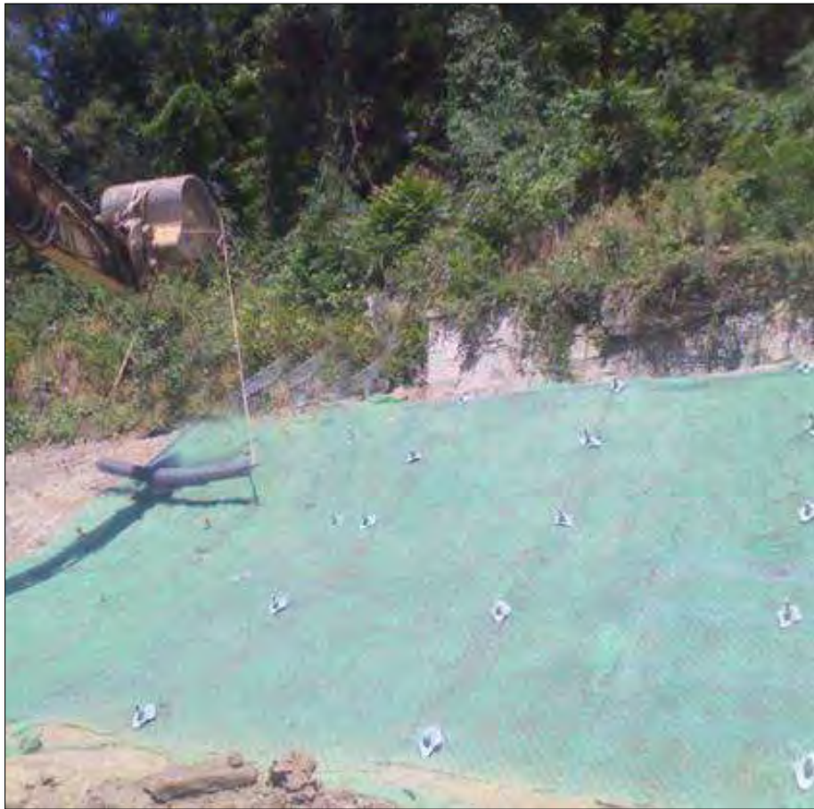
Figure 10-78 - Hydroseeded Soil Nail Slope
