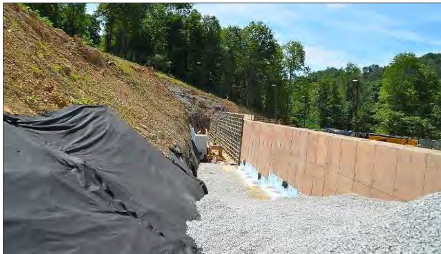
Figure 10-43 - Concrete Gravity Wall Construction, Landslide Repair
