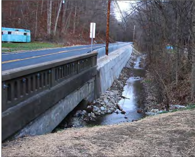
Figure 10-48 - Jumbo Block Slope Repair in Washington County, PA (PennDOT District 11)
