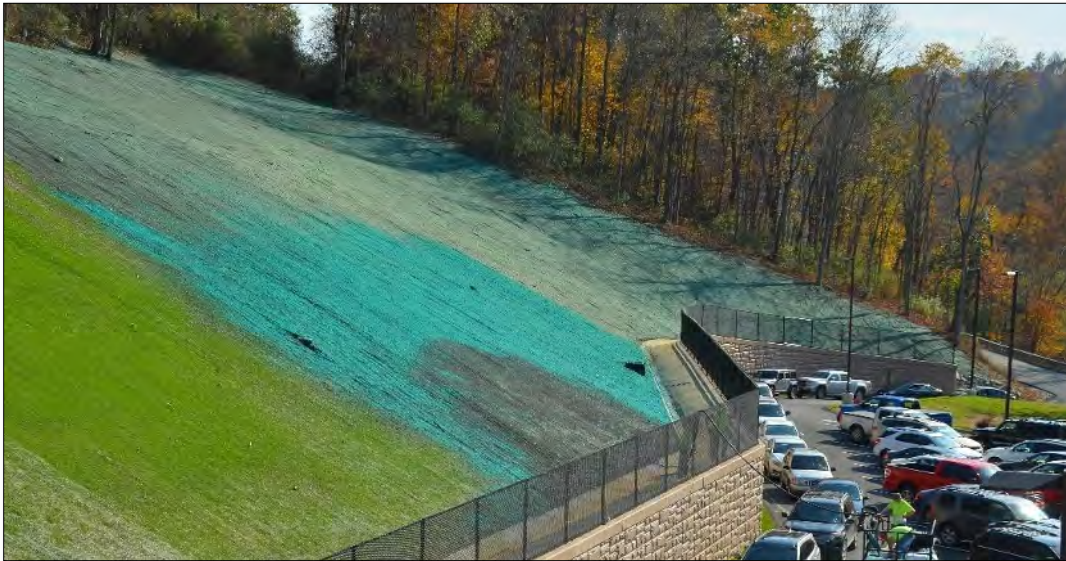
Figure 10-29 - Turf Reinforcement and Hydroseed to Installed Repair and Stabilize Slope
