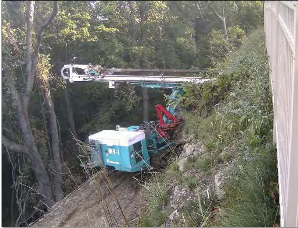
Figure 10-101 - Drilling to Install Horizontal Drains, Allegheny County, PA
