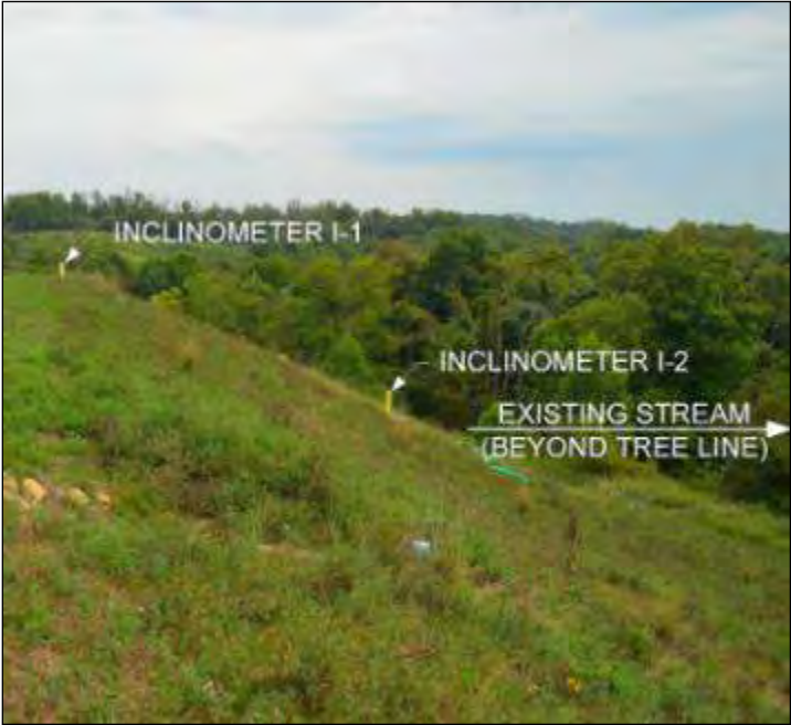
Photograph 1. Typical Section of Southeastern Slope; inclinometer locations visible
