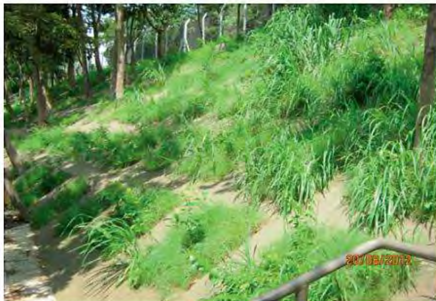
(b) Completion of soil nails and grillage construction.
