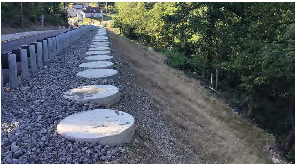
Figure 10-60 - Tangent Piles (PennDOT District 11)
