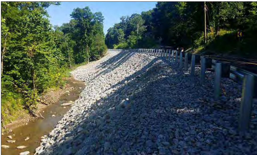
Figure 10-30 - Rock Slope Armoring
