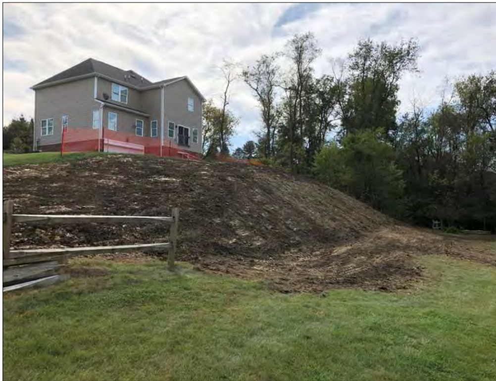
Figure 10-112 - Regraded Slope
