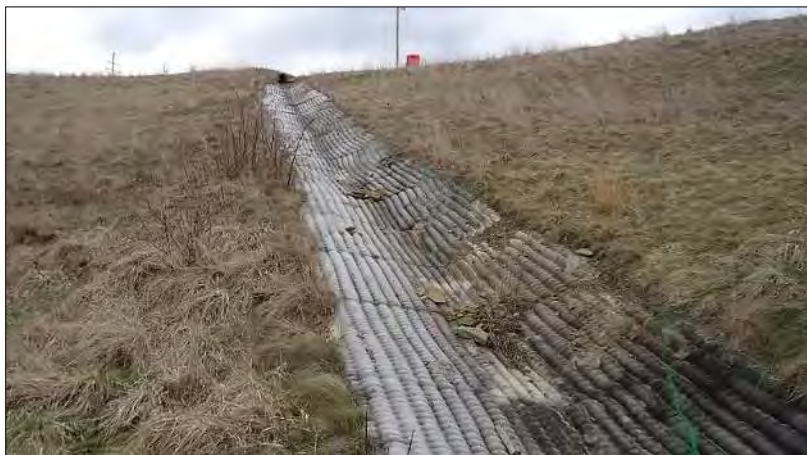
Figure 10-91 - Fabriform Lined Ditch
