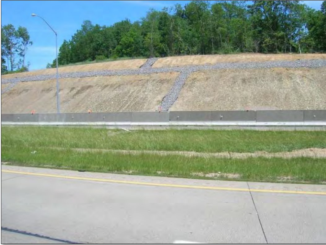
Figure 10-100 - Finger Drains on Slope
