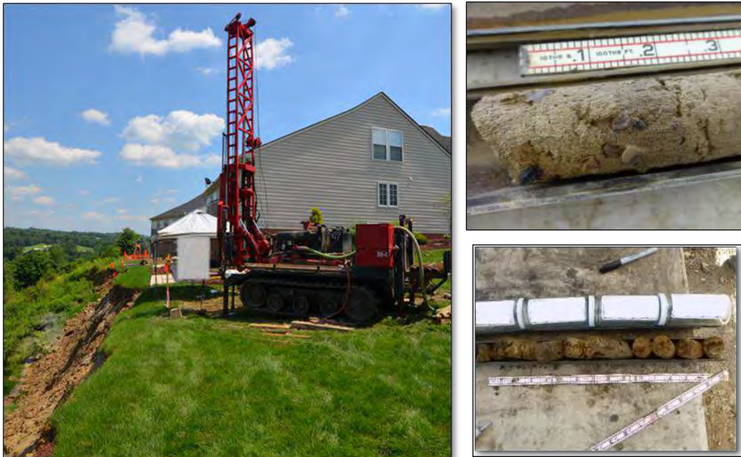
Figure 4-9 - Test boring investigation using hollow stem augers and split spoons
