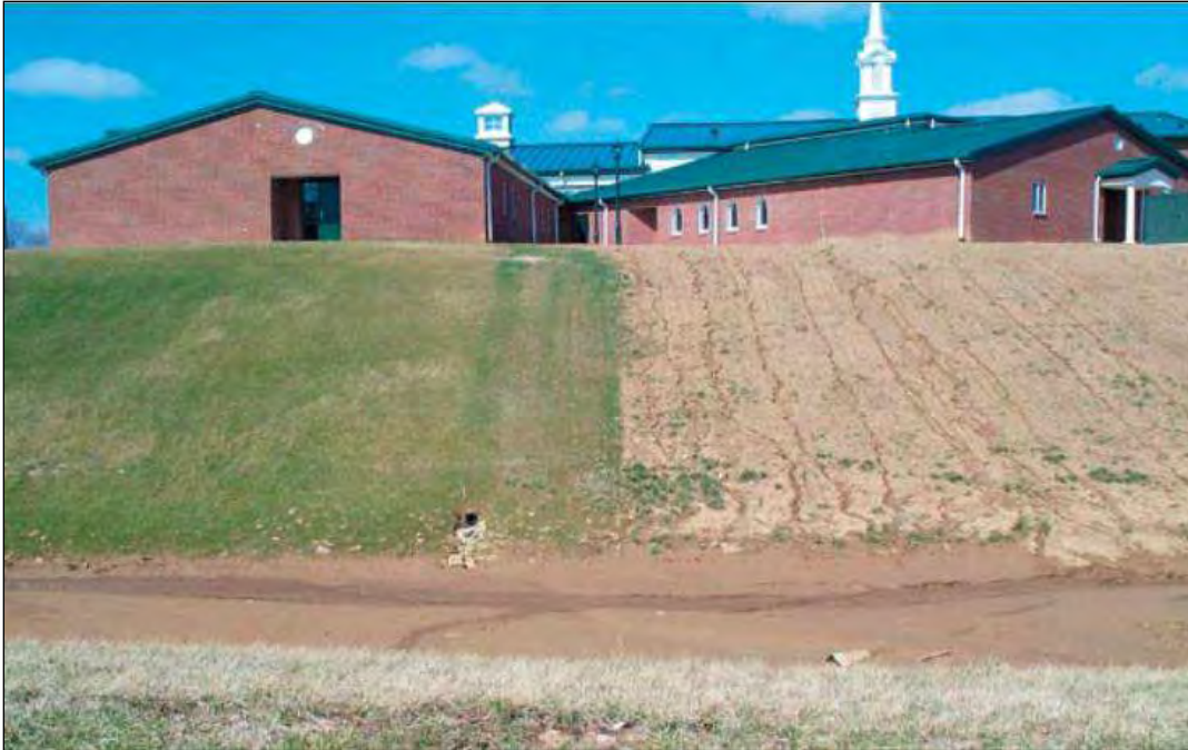
Figure 8-10 - The value of seeding/vegetation on a slope: the left (seeded) section shows almost no erosion; right side rills are quickly becoming gullies [82]
