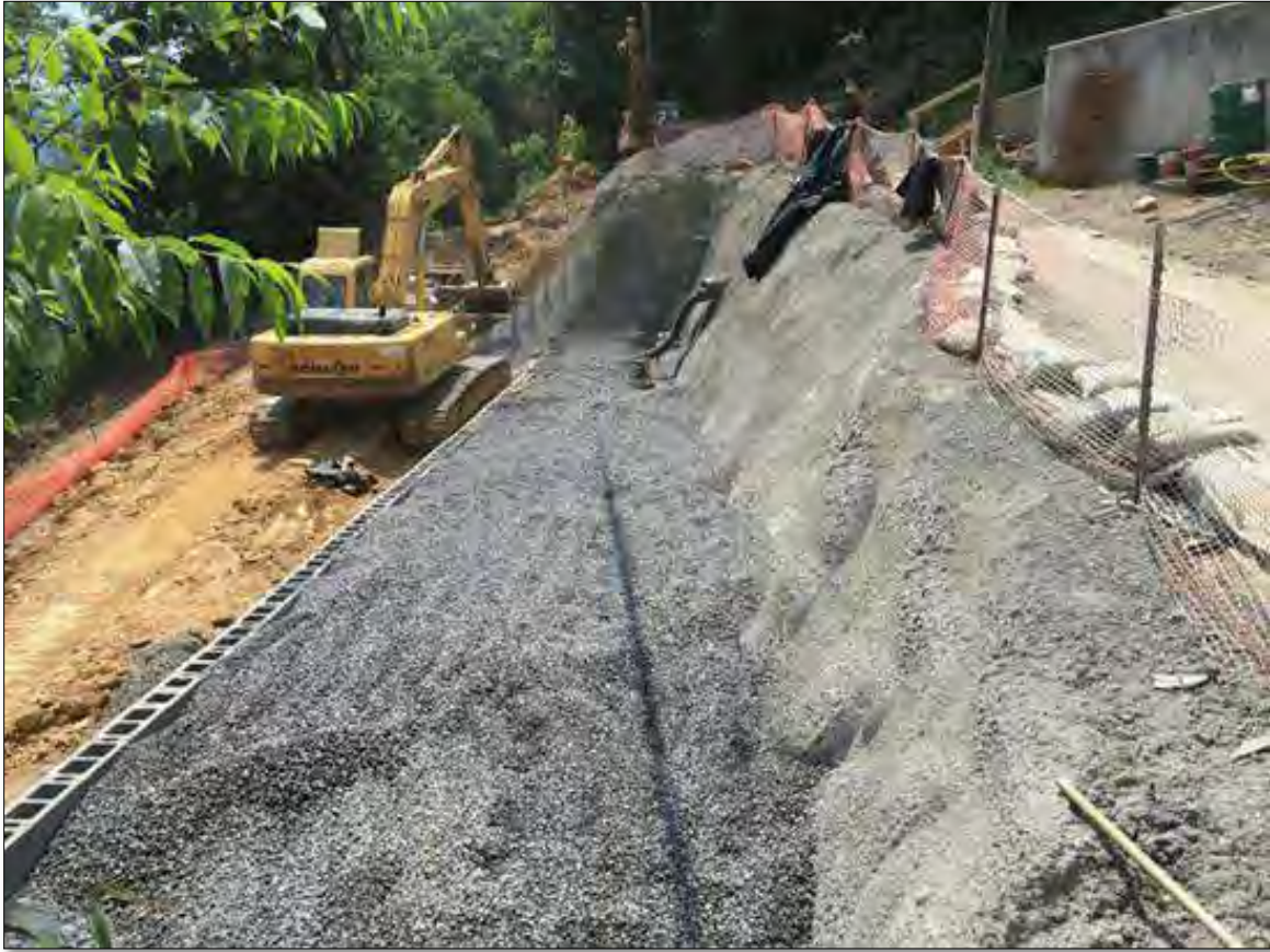
Figure 10-79 - Shotcrete and Modular Block Installation in Front of Soil Nail Slope
