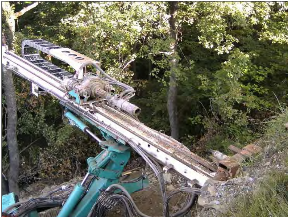
Figure 10-102 - Drilling to Install Horizontal Drains, Allegheny County, PA
