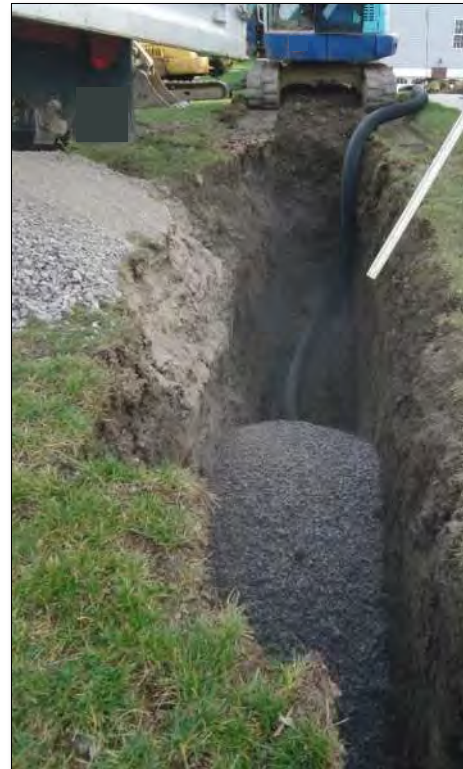
Figure 10-93 - Interceptor (French) Drain
