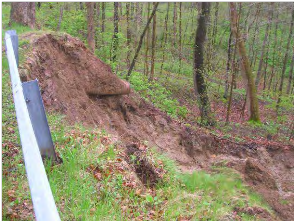
Figure 4-4 - Landslide triggered by saturated soils and erosion gullies; drainage pipe concentrating water on the slope was observed during reconnaissance
