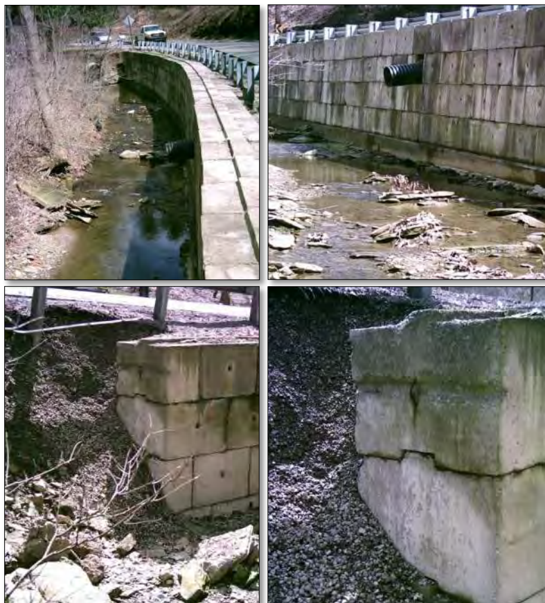
Figure 10-49 - Modular ("Jumbo") Block Wall
