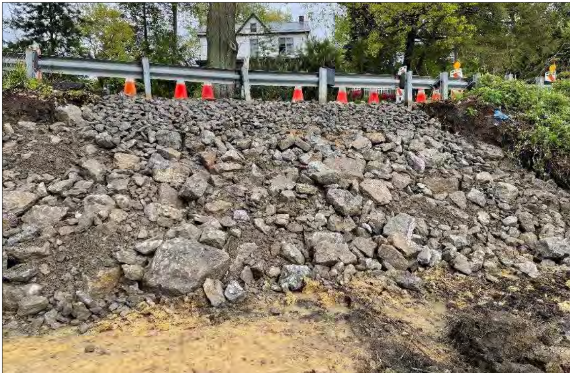
Figure 10-11 - Rock-Fill Buttress Example – Completed Repair Looking Upslope from Toe
