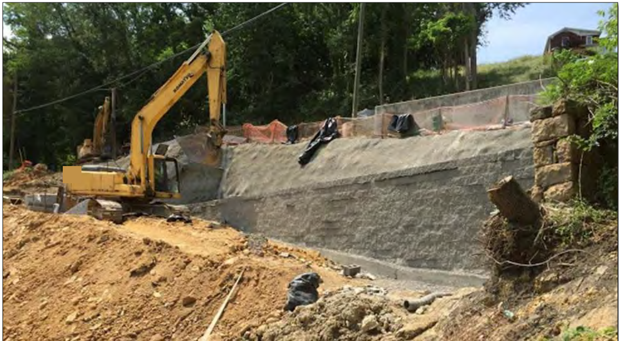
Figure 10-80 - Shotcrete and Modular Block Installation in Front of Soil Nail Slope
