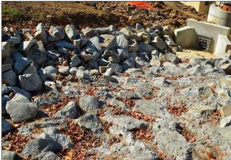
Figure 10-90 - Grouted Rock-Lined Ditch
