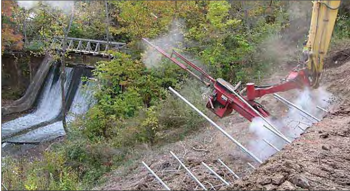
Figure 10-81 - Soil Nail Launcher [13]
