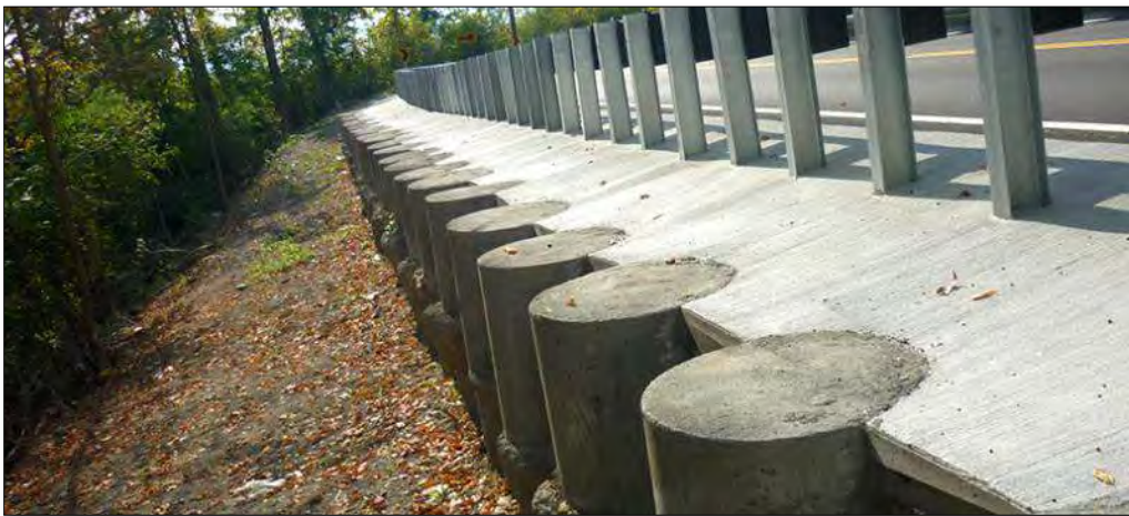
Figure 10-59 - Tangent Pile Wall Supporting Roadway Shoulder [23]
