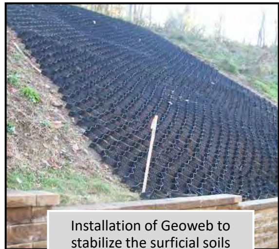
Figure 8-11 - Geoweb installation
