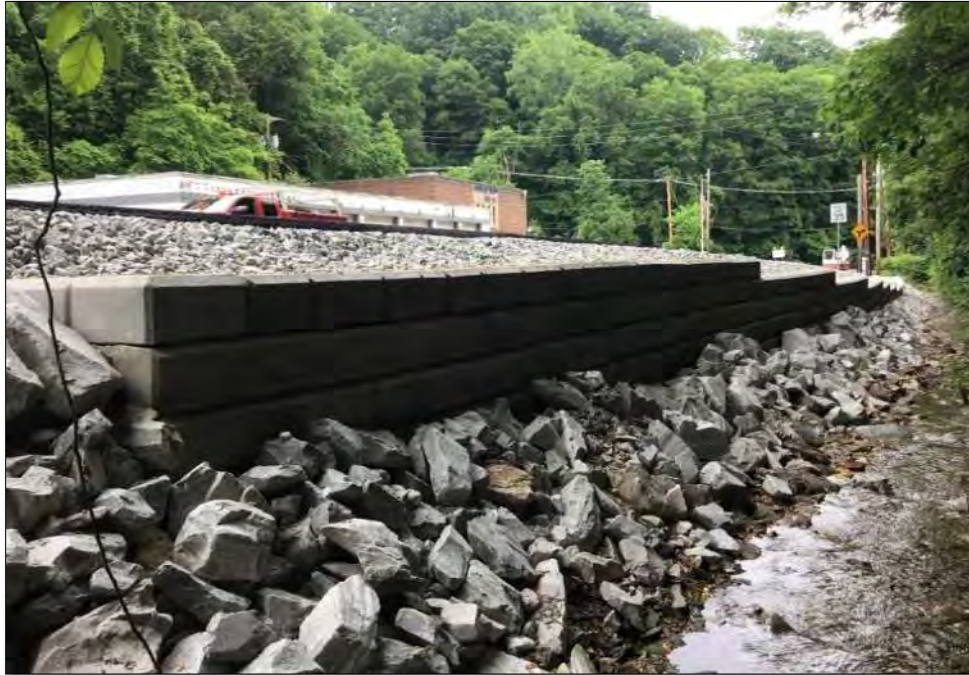
Figure 10-52 - Durahold Wall (PennDOT District 11)
