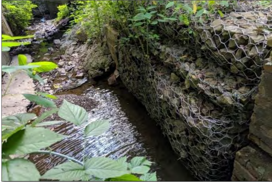
Figure 10-44 - Gabion Wall
