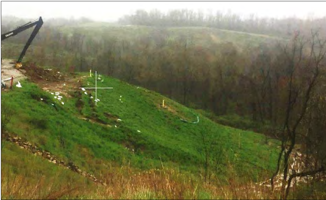
Figure 10-107 - Partial Unloading of Slide Mass
