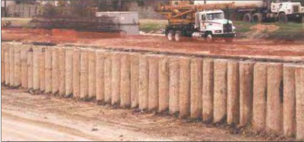
Figure 10-58 - Tangent Pile Wall [48]
