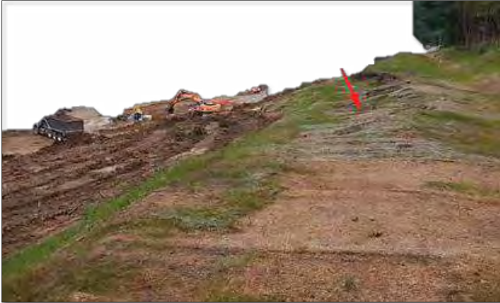
Figure 10-27 - Head Scarp of Carpet Slide
