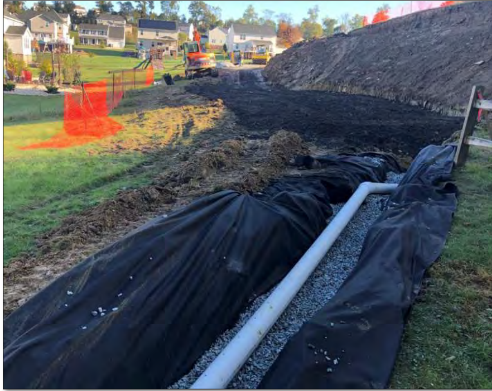
Figure 10-111 - Drain Installation in Toe Key
