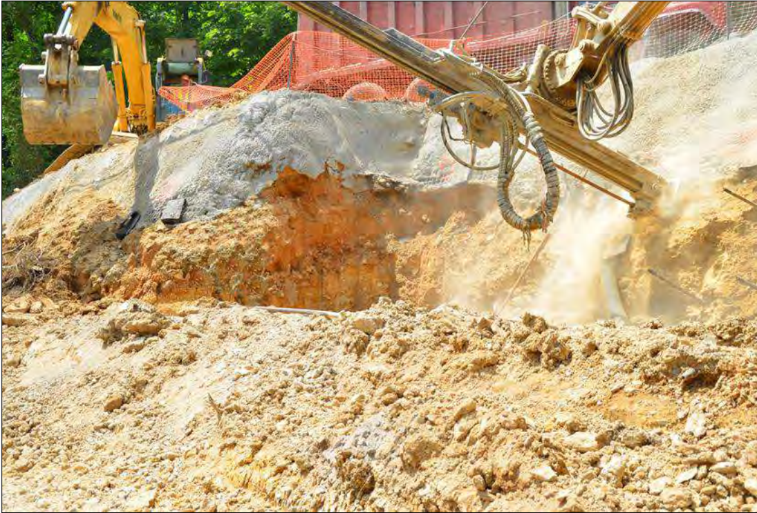
Figure 10-75 - Soil Nail Drilling
