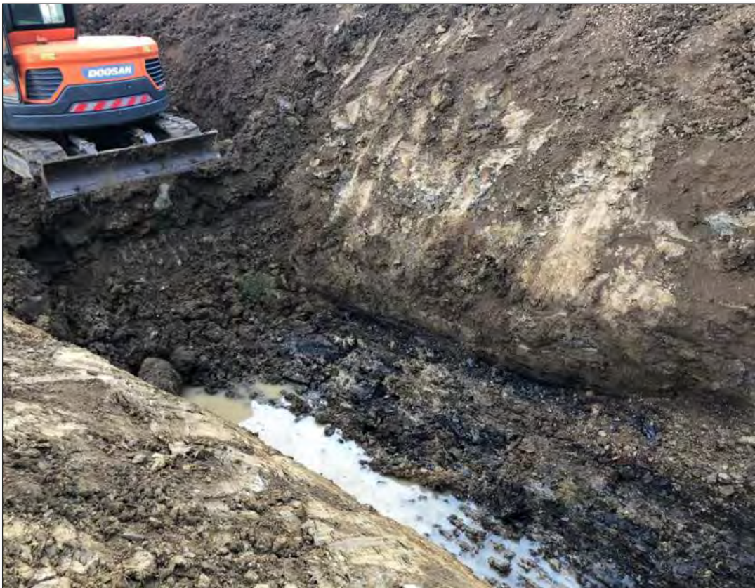
Figure 10-110 - Toe Key Excavation
