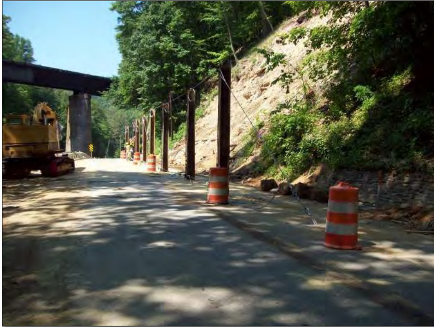
Figure 10-115 - Debris Flow Fence Installation
