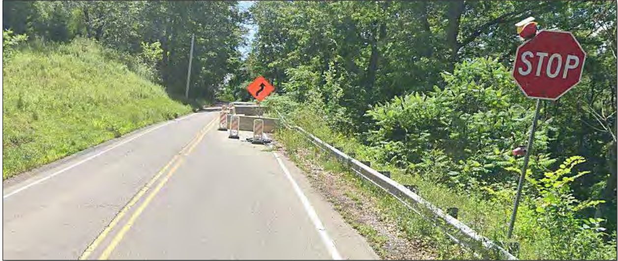
Figure 10-2 - Relocation Example Extended Term Lane Closure
