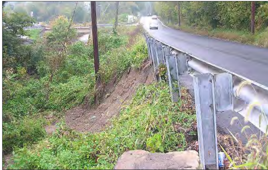
Figure 10-53 - Landslide Area, Before Stabilization with a Soldier Pile and Lagging Wall
