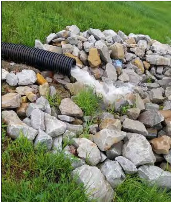
Figure 8-8 - Rip Rap protection at drain outlet (left)
