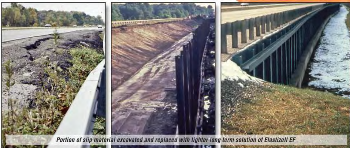
Figure 10-106 - Elastizell for Landslide Repair [36]
