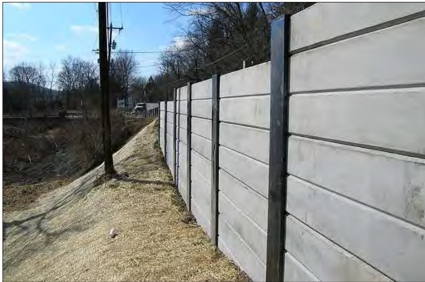
Figure 10-54 - Landslide Area, After Stabilization with a Soldier Pile and Lagging Wall
