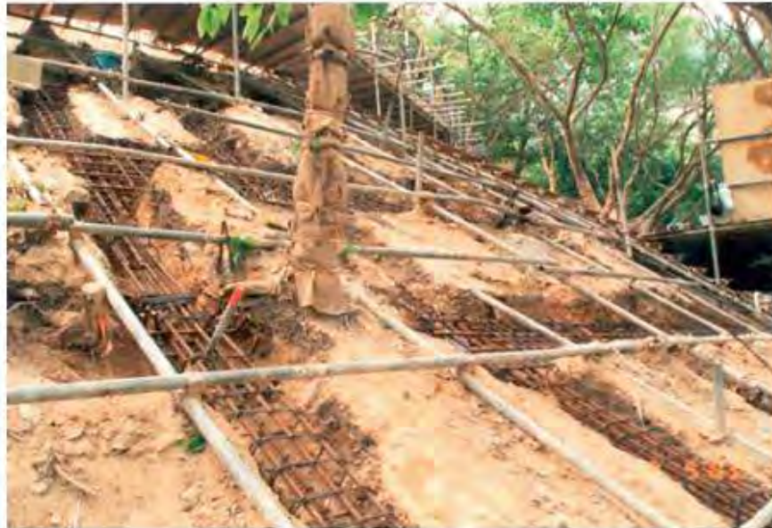
(a) Construction of soil nails and grillage.
