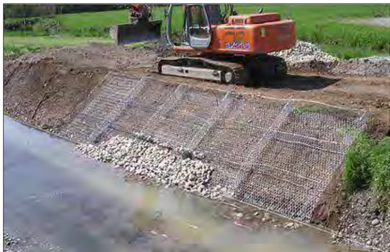
Figure 10-37 - Reno Mattress Installation [55]
