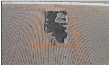
Partial Depth Repair
