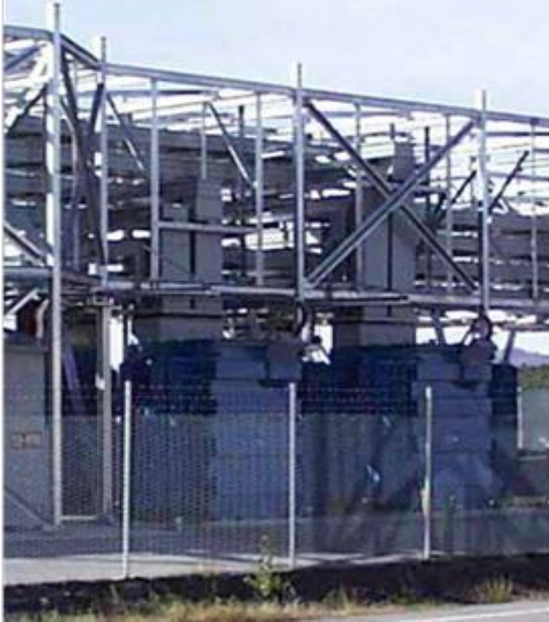
Conventional 60Hz Power Transformer (60Hz, 100kV, 20A RMS, >30 tons)
