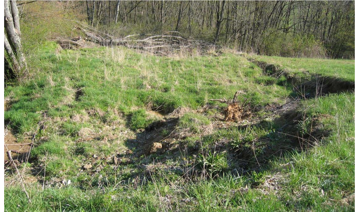
Landslide over the Cumberland Mine after longwall mining, Greene County, 2005
