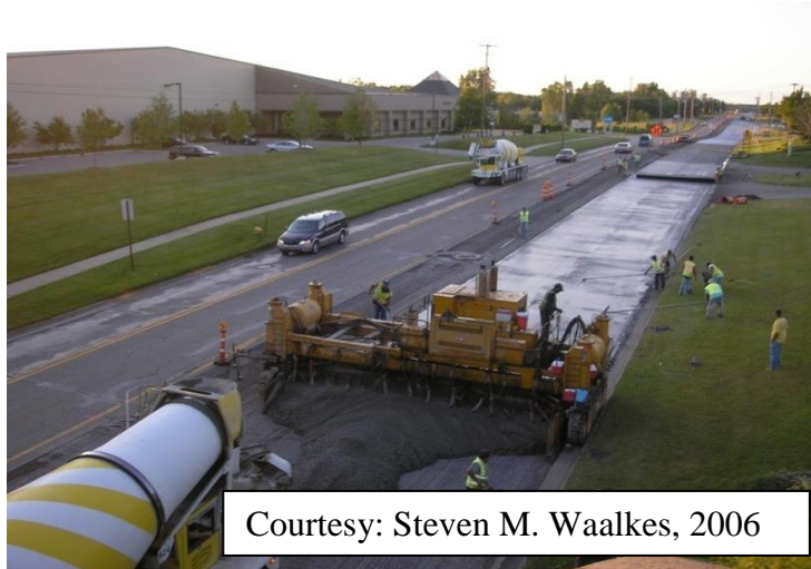
Figure 47: Condition of the original HMA layer at the time of construction.
