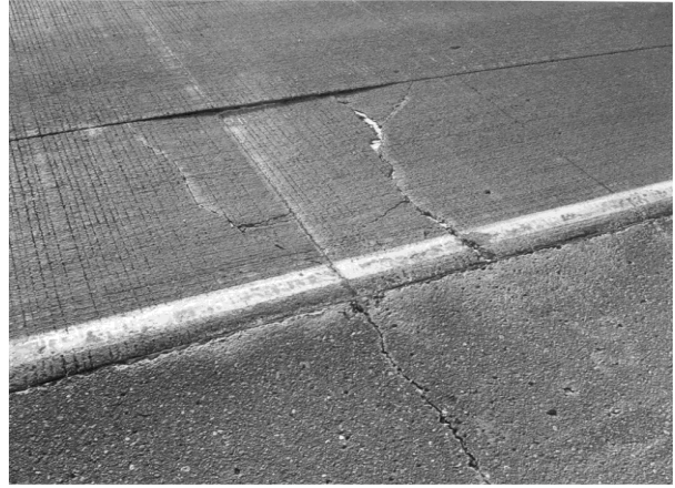
a.) Development from corner cracks. b.) Development independent of other cracking.
