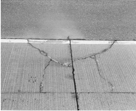
a.) Development from corner cracks. b.) Development independent of other cracking.
