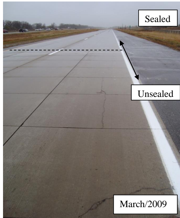
Figure 30: Difference in the amount of water infiltrating the surface for the sealed and unsealed sections.
