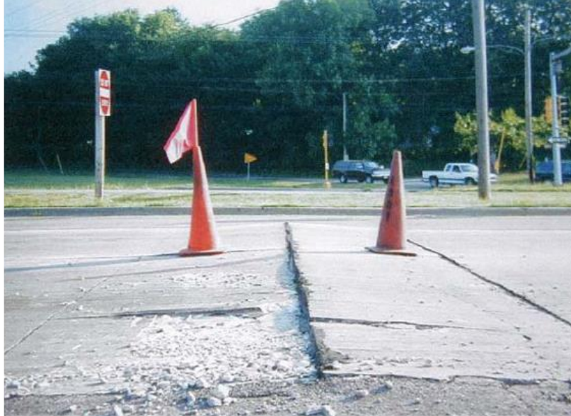
Figure 46: Blow up of the UTW slabs (Winkelman, 2005).
