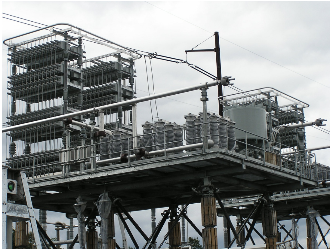
Redundant Fiber Optic Columns on Platform
