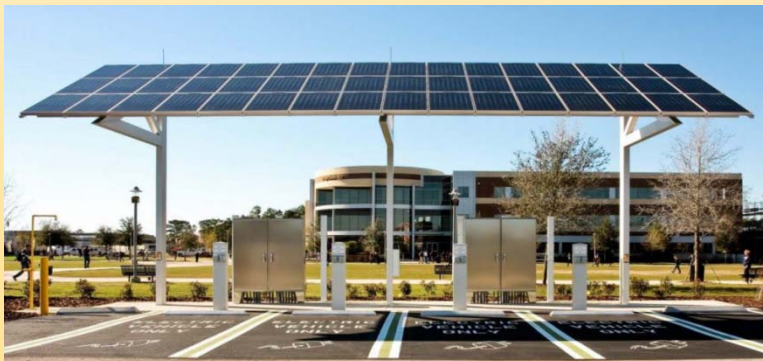
Electric Vehicle Charging Station [1]
