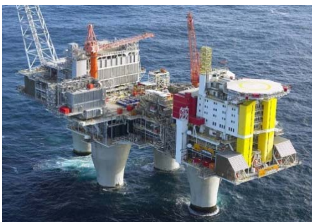
Troll 1 & 3 80+80 MW HVDC Power from shore 2005 / 2015
